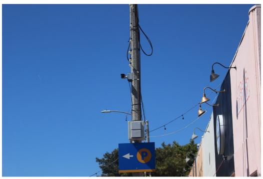
A camera aimed at a zero emission loading zone within the City of Santa Monica's pilot area. These cameras were sited and installed by Automotus for monitoring purposes rather than for enforcement.
