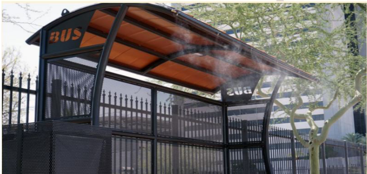
Fig 4: Misted Bus Shelter in Phoenix, Arizona
